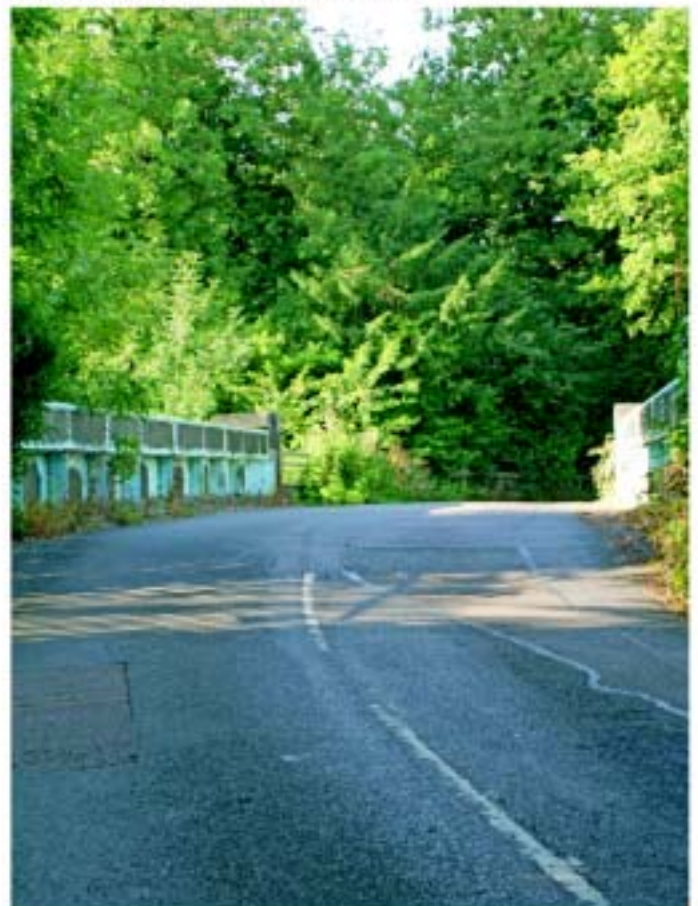
Mill Lane Bridge
